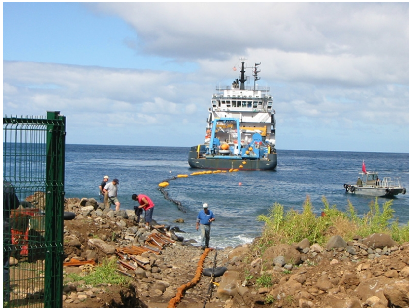
Laying cable for hydroacoustic stations (CTBTO)
